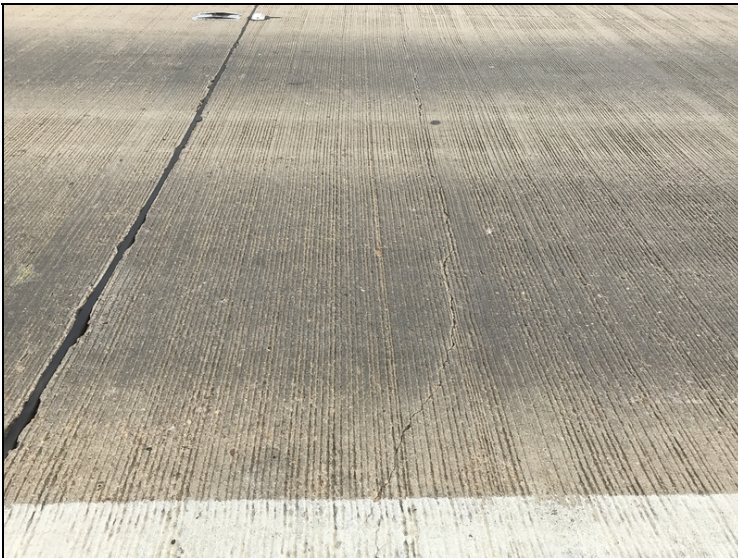
Approach slab cracks
