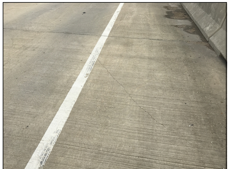
Typ top flange cracks near corners
